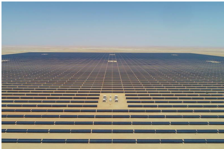
Amin solar power plant
