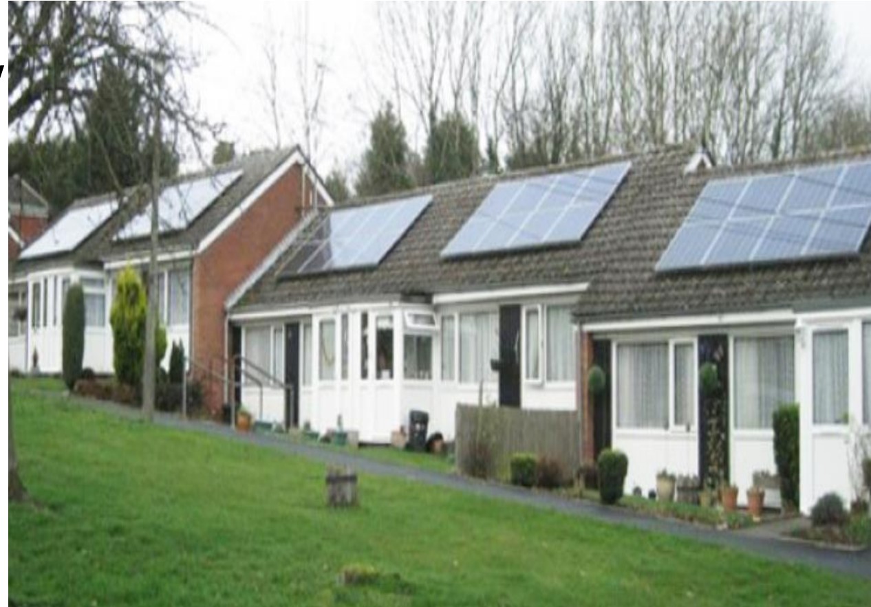
Solar panels on council housing in Warwickshire
